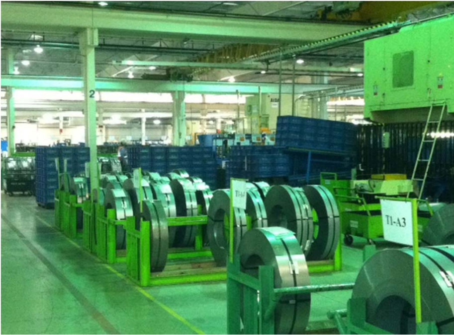
Pre-Installation HID Fixtures
